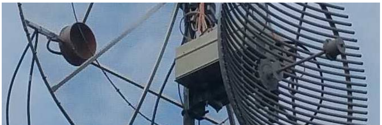
HA5UA - back side of 1.5m mesh dish 3.5GHz 80cm grid
